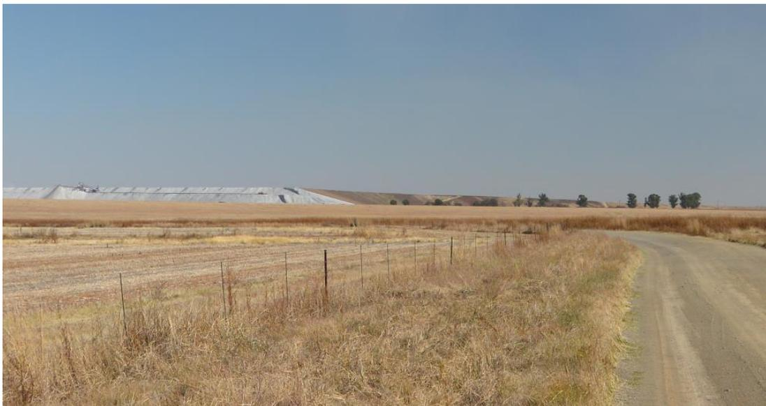
**Figure 8: Rehabilitation of the ash disposal facility by vegetating slopes increase the visual absorption capacity of the feature – noticeable on the right section of the photograph.**
